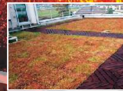
EcoSedumPack - zielony dach
